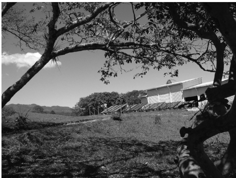
Figure 2.1. Solar-hybrid coffee drying facility in Subirana, Honduras. Panels in foreground collect thermal energy, which is circulated through drying towers located in the building behind.
